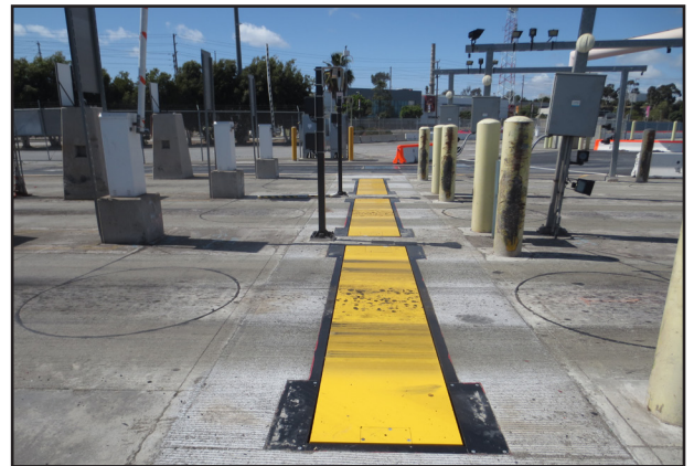
Low-Speed Weigh-In-Motion (LS-WIM) scales provide excellent accuracy with a high-quality, durable scale.
