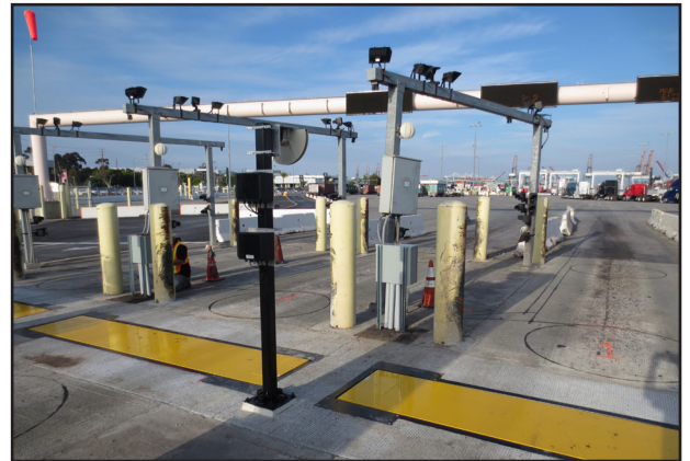
Automate gate processes, with Gross Vehicle Weights, vehicle ID, images, and cargo profile incorporated into a WIM system.
